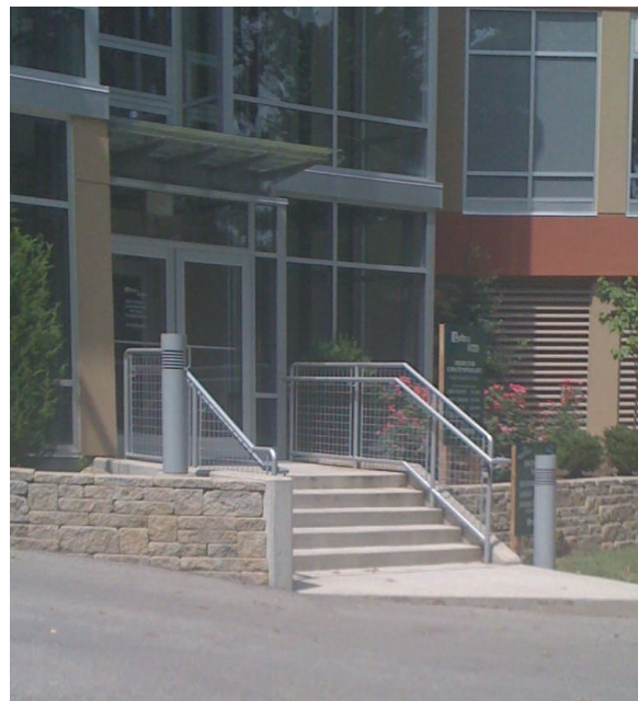
The main entrance of The Lofts in Oakley has steps that make it impossible for someone in a wheelchair to enter. The Fair Housing Act requires that multifamily buildings constructed after 1991 be accessible.
